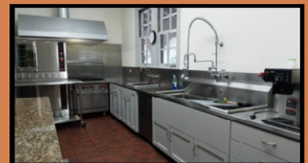
2018 Crespi Hall Renovation
