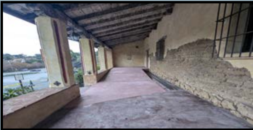
THE RAMP TO THE BLESSED SACRAMENT CHAPEL HAS BEEN INSTALLED
